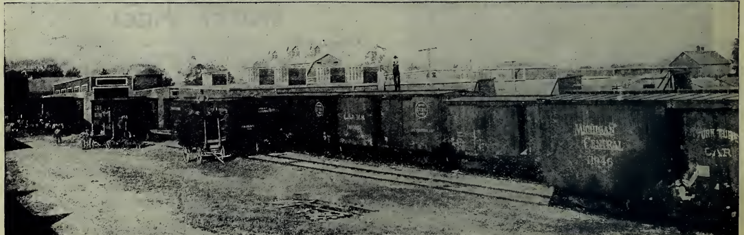
Views of part of the Greenhouse equipment, propagating frames, barns, side track and shipping facilities of The Storrs & Harrison Company, Painesville, Ohio
